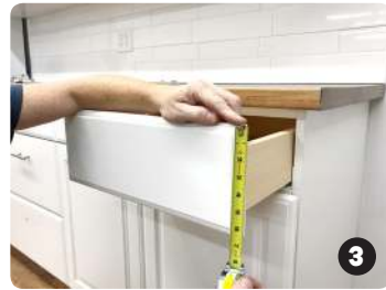
Measure side of drawer for center. Position hardware where you like
