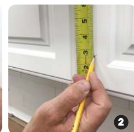
2 Measure from bottom mark position with pencil
