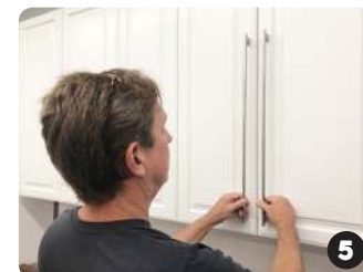
Position hardware by hand to find where you like it and mark position of bottom hole
