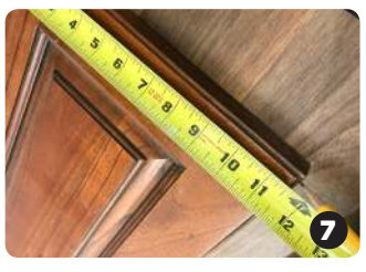
7 Measure height of drawer use half that number for center
