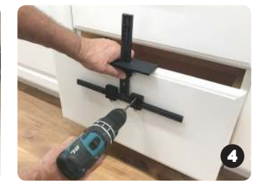
Center on drawer and drill holes
