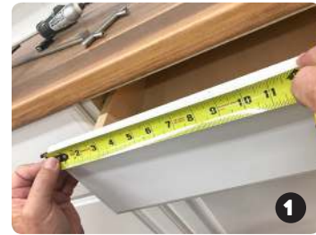
Measure width to find center
