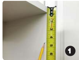
Mark center of two hinge holes
