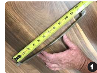
Measure hardware hole spacing
