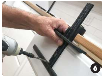
Drill hole using fixed center drill bushing
